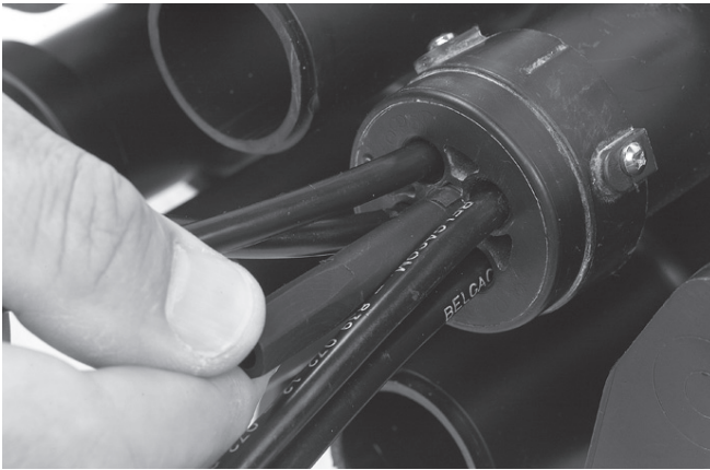
3.2.1.7 Tighten the trigger till it butts up with the flange. The spring should be hidden after tightening.
